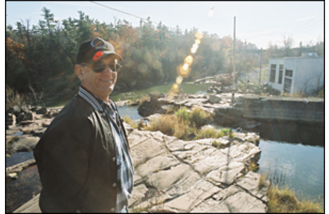
Photo: Robert Fleming International Research Inc. / Dick Allen maintained the Kingston Mills hydroelectric power station for 35 years before retiring two years ago
