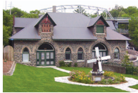
Bracebridge Falls Generating Station, Bracebridge, ON
